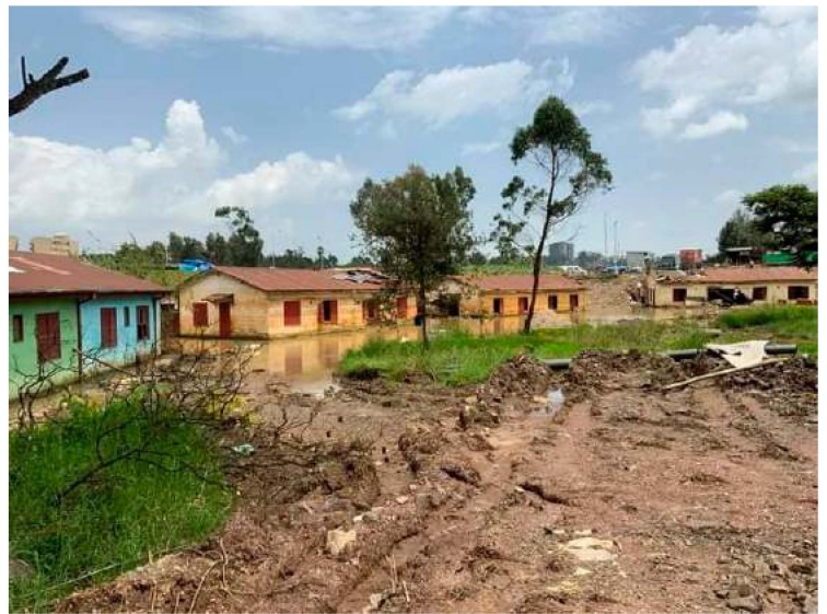
Flood damage at the Mekane Yesus Seminary
