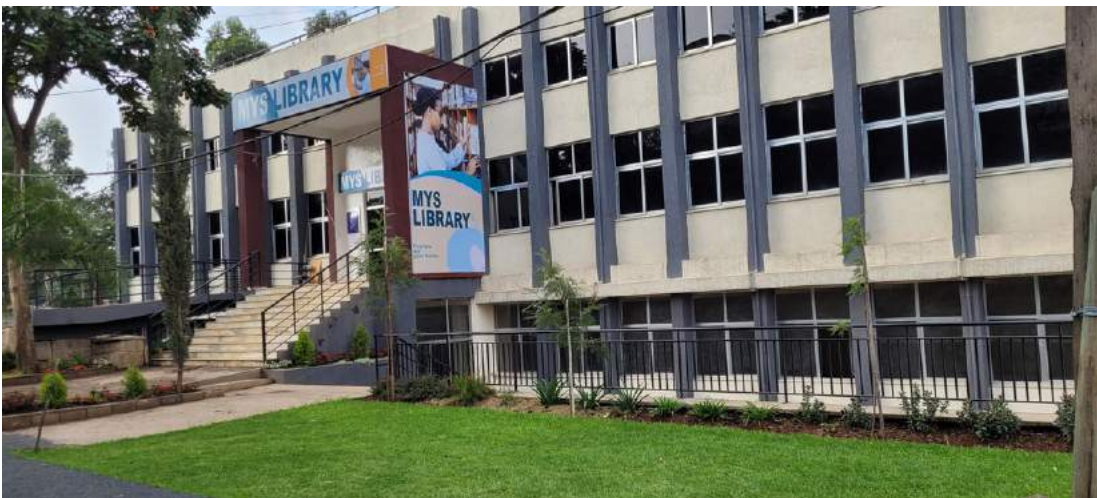
Mekane Yesus Seminary library cleaned up from the flood damage
