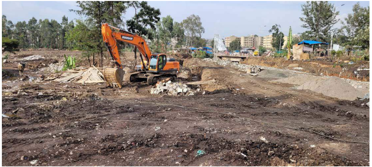
Cleanup of the flooded area continues a year later
